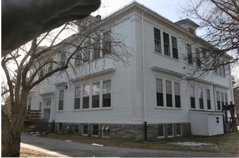
Photo 2. East and north elevations.
