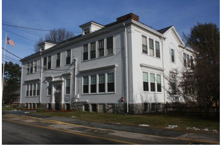
Photo 1. West and south elevations.
