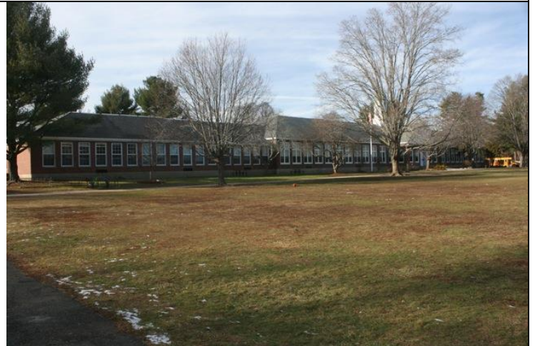
South Wing (L) and Original Building (R): facade/east elevations.
