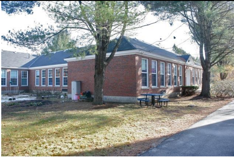
South Wing: view SE (southwest elevation on right).
