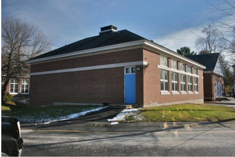
Cafeteria Wing: N and W elevations.
