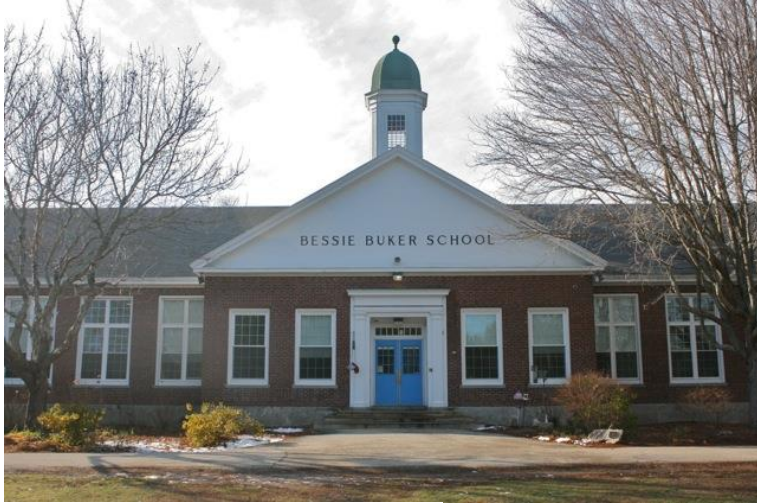
Original Building: facade (east elevation)
