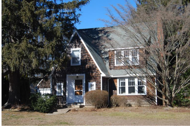
7 Porter Street, view looking northwest.
