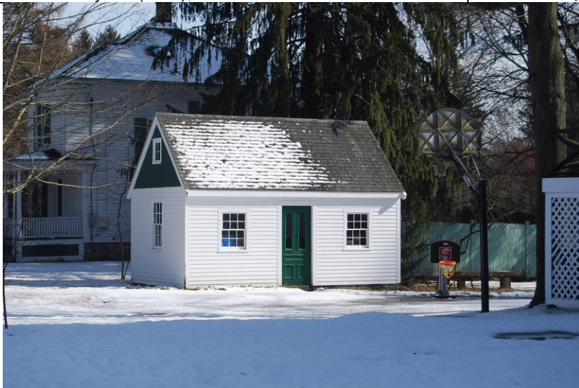
Photo 4. Shed. West (main) and north elevations.
