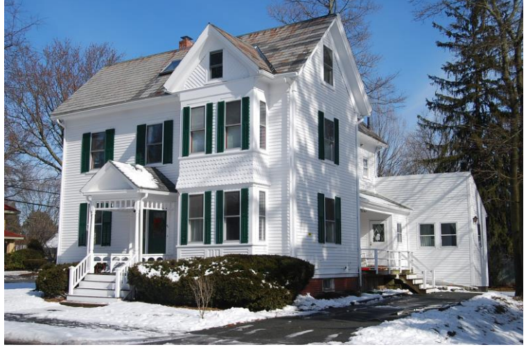
Façade (west) and south elevations.
