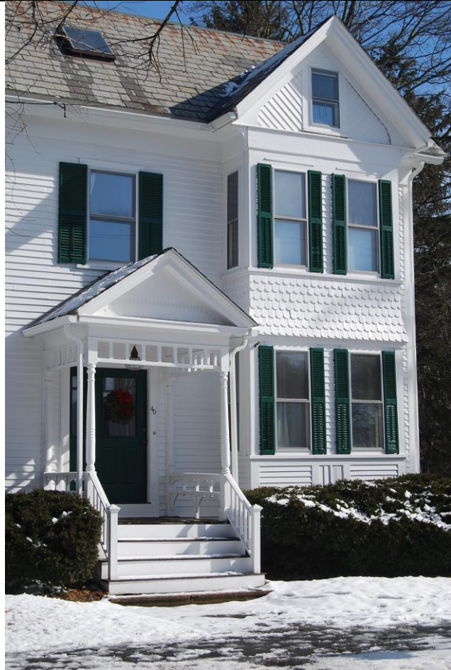
Photo 2. Façade (west), detail.
