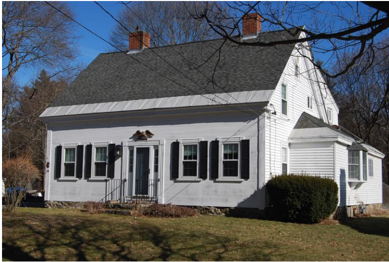
Façade (west) and south elevations.
