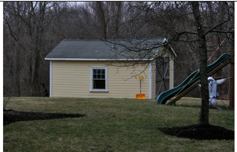
Photo 3. Garage. East and façade (north) elevations.
