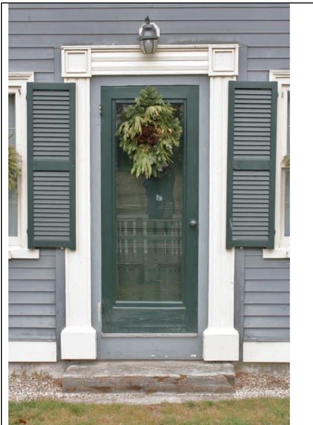
Photo 2. Façade (west), entrance detail.
