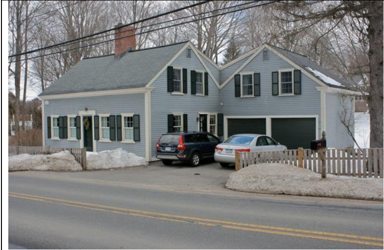
Façade (west) and south elevations.
