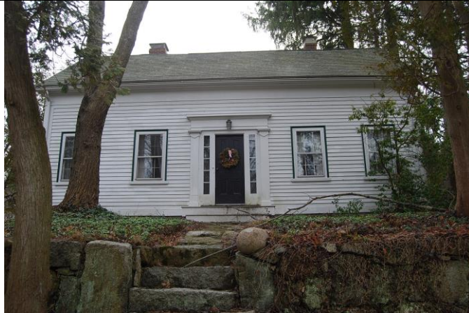
Photo 2. Façade (northeast) elevation.
