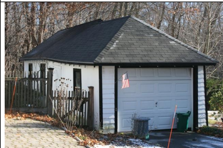
Photograph 11. 25 Friend Court garage
