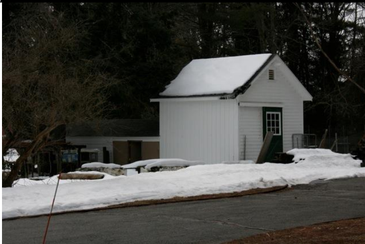
Photo 4. Outbuilding 1: East and north elevations.
