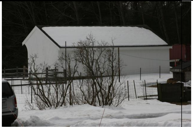
Photo 5. Outbuilding 2: East and north elevations.
