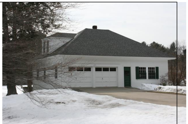
Photo 3. Garage. East and north elevations.
