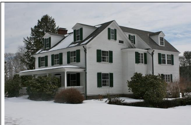
Photo 2. Façade (north) and west elevations.
