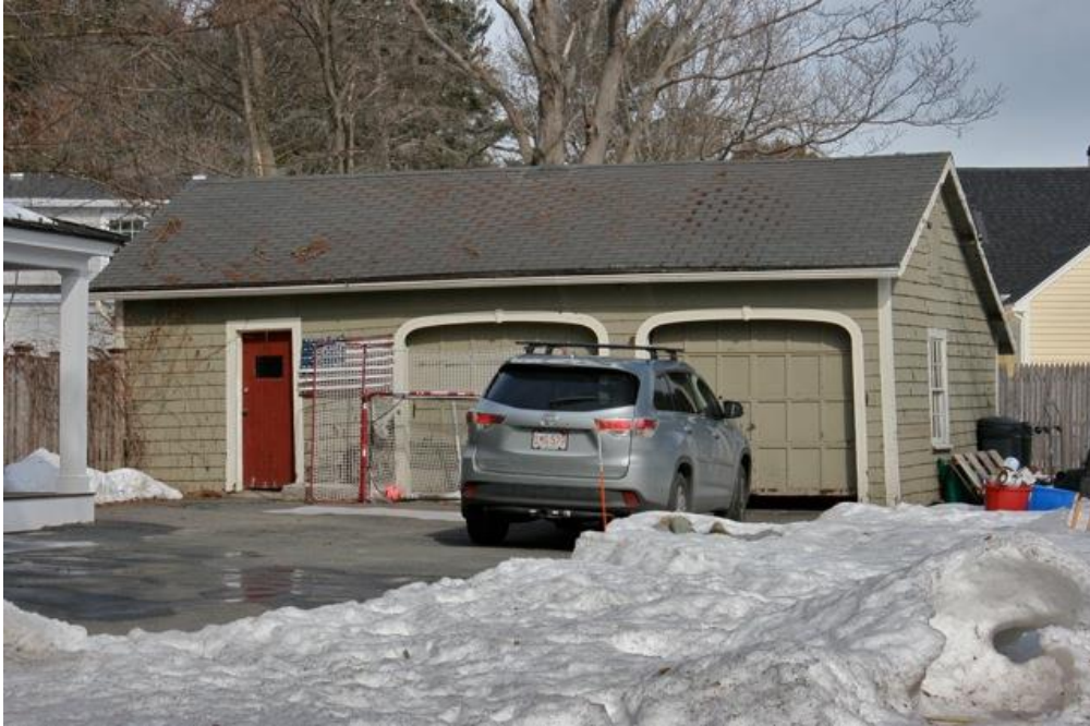
Garage. West (main) elevation.
