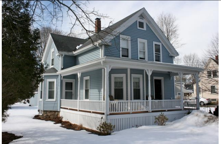
Façade (north) and east elevations.
