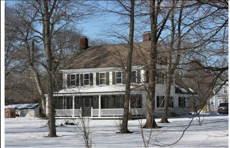
Façade (south) and east elevations.
