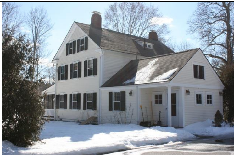
Photo 2. East and north elevations.
