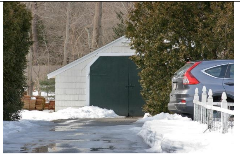
Photo 3. Garage. Façade (east) elevation.
