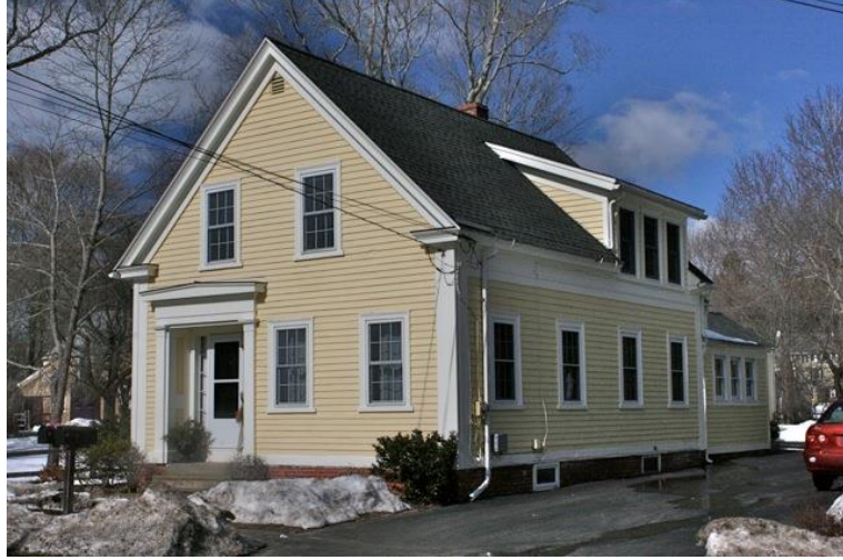
Main (South) and east elevations.
