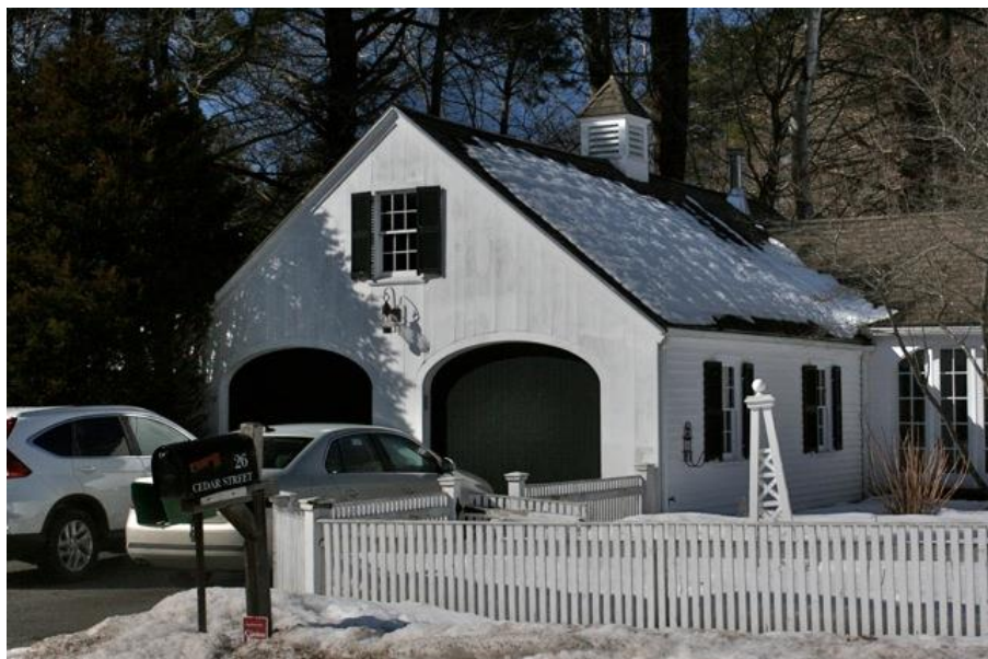
Outbuilding. South and east elevations.
