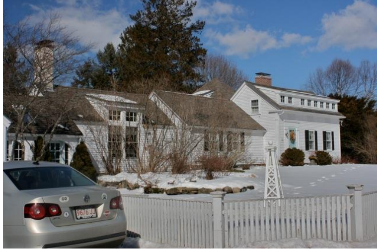
Façade (south) elevation.
