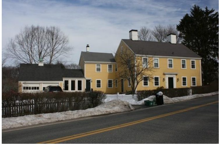
Façade (south) elevation.
