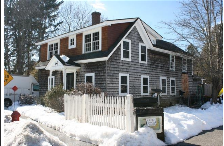
Façade (east) and north elevations.
